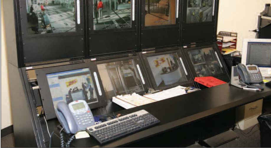
DHL's state of the art control room video wall consists of eight monitors with two monitors split into quad screens, all controlled from a single Workstation PC using OnSSI's NetSwitcher touch-screen, dynamic map-based interface.
